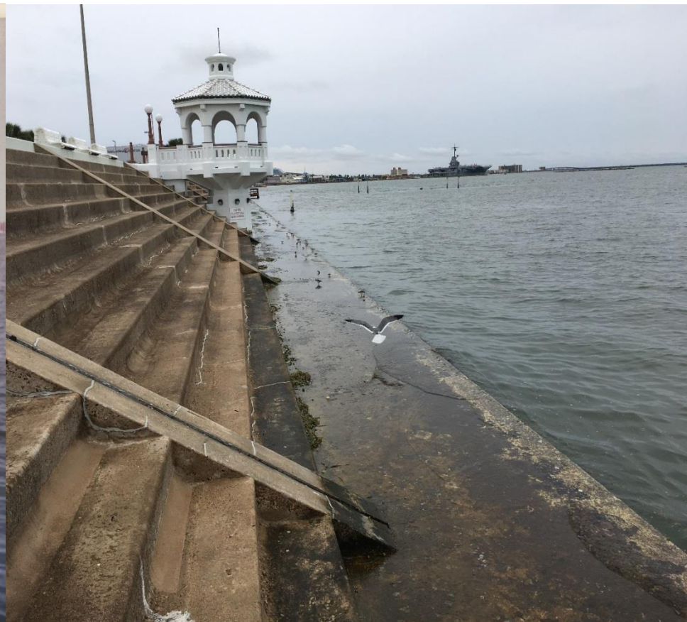
After Seawall Reconstruction (2005) New Marine Growth at Same Location 11-10-2016 High Tide
